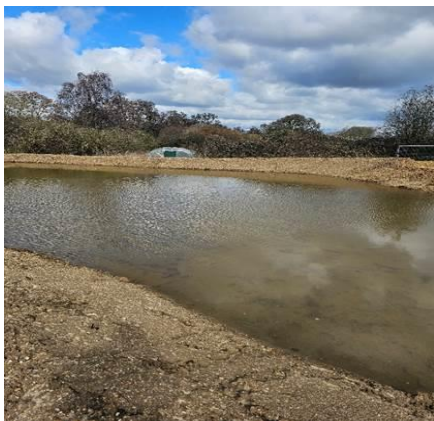
Figure 4 - Clay Lined Bed ready for Reed Planting
