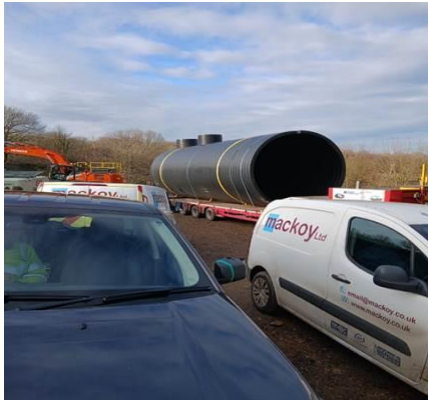
Figure 3 - Delivery of settlement tank
